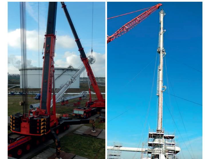
Lifting of the first section of the stack
